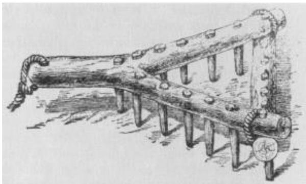
Figure 1.2 Home-made harrow similar to that used for “mullensing” or “Yankee grubbing” in the Mallee in the nineteenth century
