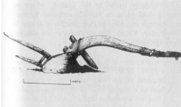
Figure 1.1 Heavy wooden breaking plough used for breaking up virgin country in the early nineteenth century
