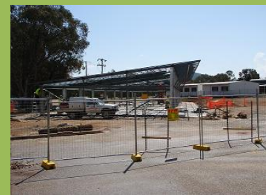
New Residences – Thurgoona Under Construction
