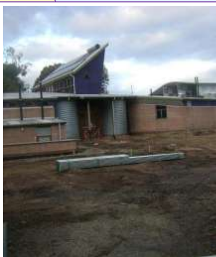
Construction is starting on the Gums "G" Bar project at Thurgoona
