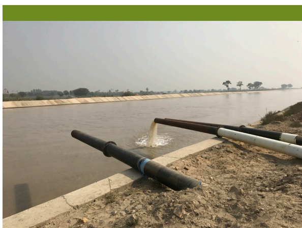
Seepage from the main canal had affected nearby farms with raised water table. Pumping water back into the canal has helped replenish productivity. Nawabshah in Sindh province.
